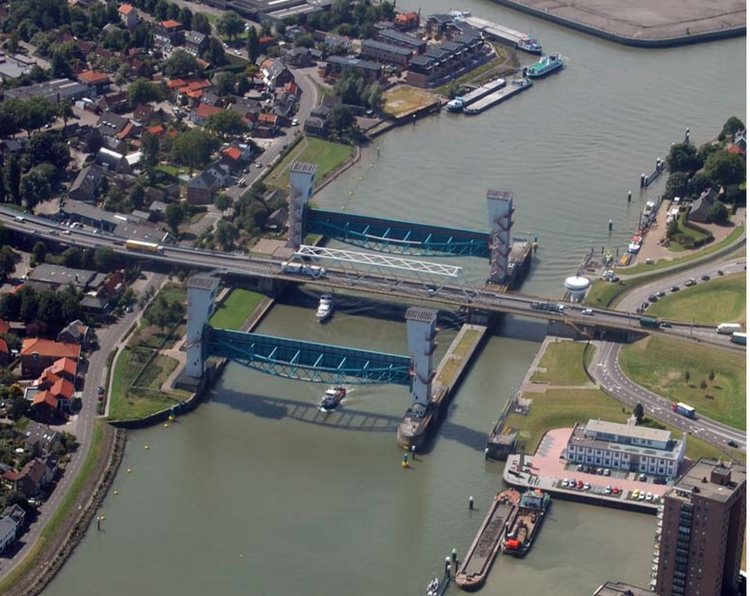
First storm barrier completed under the Delta Works: the Hollandse IJsselkering at Krimpen aan de IJssel
